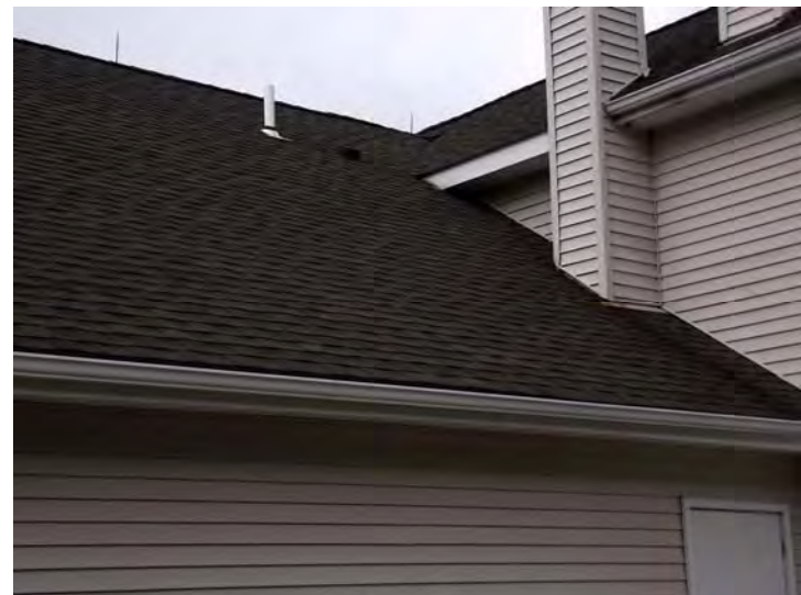
Buildings have pitched roofing covered with architectural shingles.
