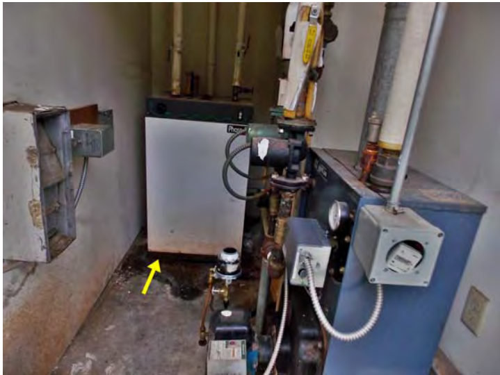
Each mechanical room contains a propane fired boiler (on right) that produces hydronic heat for space heating and DHW production. In the rear (arrow) is the DHW storage tank.
