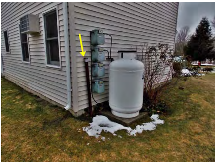
One of the fuel oil fill stations (arrow).
