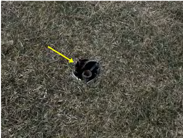
A close-up of a damaged water supply service valve enclosure.
