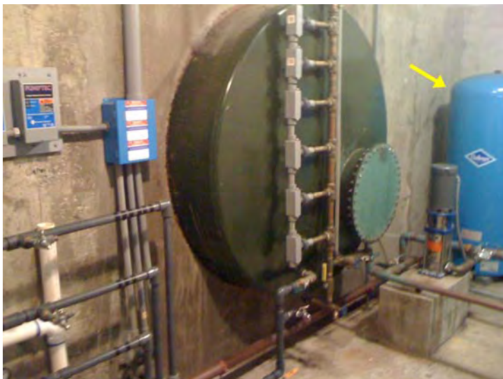
This is the 3,500 gallon domestic water storage tank. On the right (arrow) is one of the water pressure tanks.
