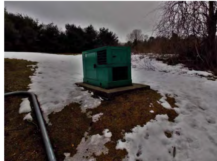
This diesel-powered generator provides emergency power for the water building.
